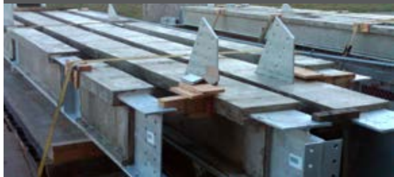
PYROCRETE 241 APPLIED OFFSITE AND TRANSPORTED TO JOBSITE.
